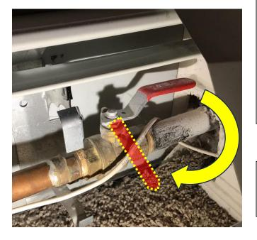
**3.** Turn the red handle 90 degrees so it is perpendicular to the pipe
