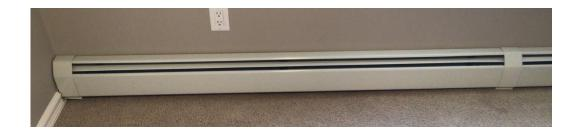
Unhook the cover clips by pulling the tab down and then towards you
